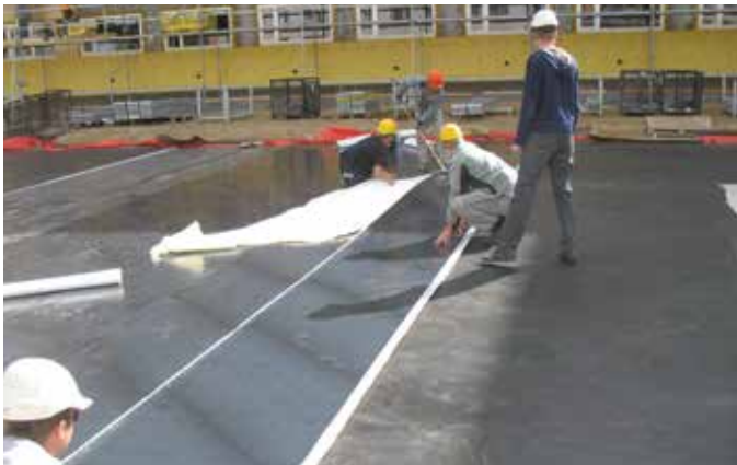
Substrate preparation
