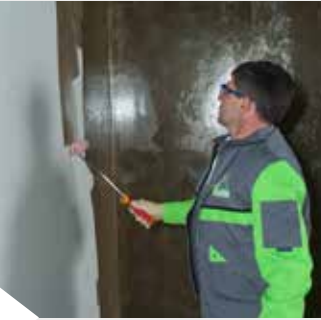
Priming the substrate
