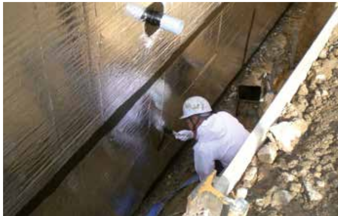
Applying the membrane
