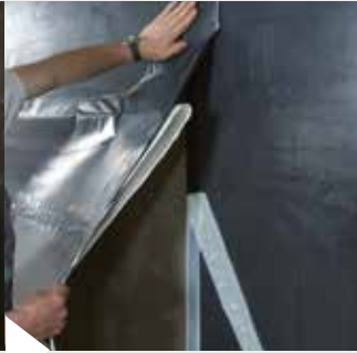
Applying the membrane
